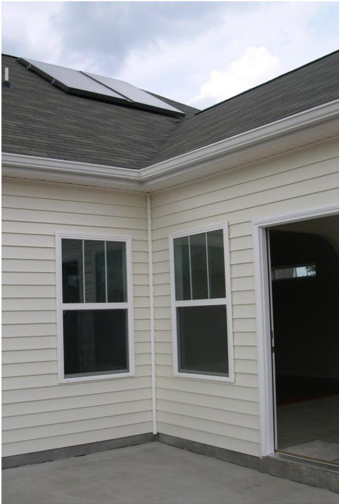
Solar panels are for installed solar hot water heater. Homeowners planned ahead and had the house pre-wired for future photo voltaic connections.
